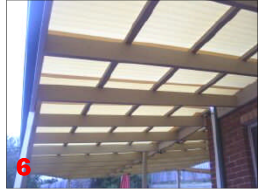
Rear covered timber pergola. (Requires Approval to be considered compliant, although it is well built and approval should only be a formality) (See photo no. 5, 6 & 7)
